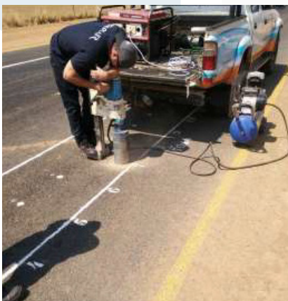
Drilling of core on prepared HVS section.
