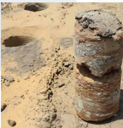
(17 January 2019) Cores drilled in the middle of the HVS test section after removal of the HVS at the end of the test after applying in excess of 7 Million E80s (more than double the design traffic loading).
